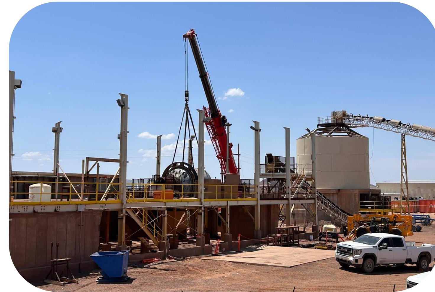
Old ball mill being removed from the process plant
