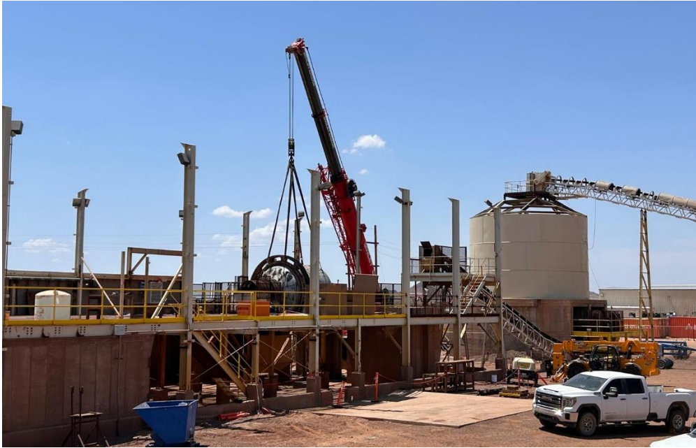
Figure 1. Historic ball mill being removed from the process plant
